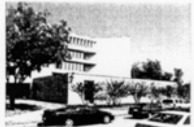
South Elevation of Existing Building
