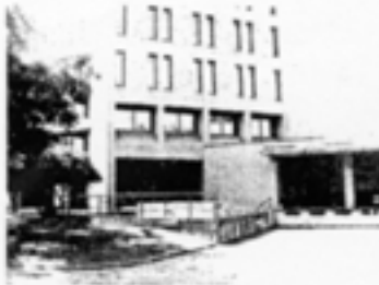
North Elevation of Existing Building
