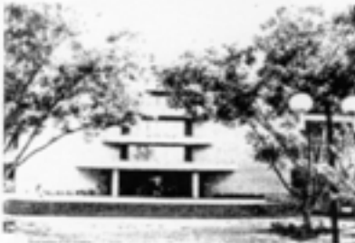
West Elevation of Existing Building
