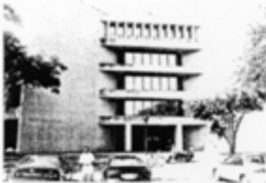
East Elevation of Existing Building
